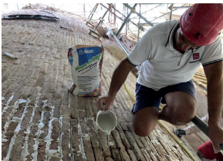
The outer faces of the ceilings were consolidated by pouring in MAPE-ANTIQUÉ F21 and then applying PLANITOP HDM RESTAURO and MAPEGRID B 250 basalt fibre mesh.
