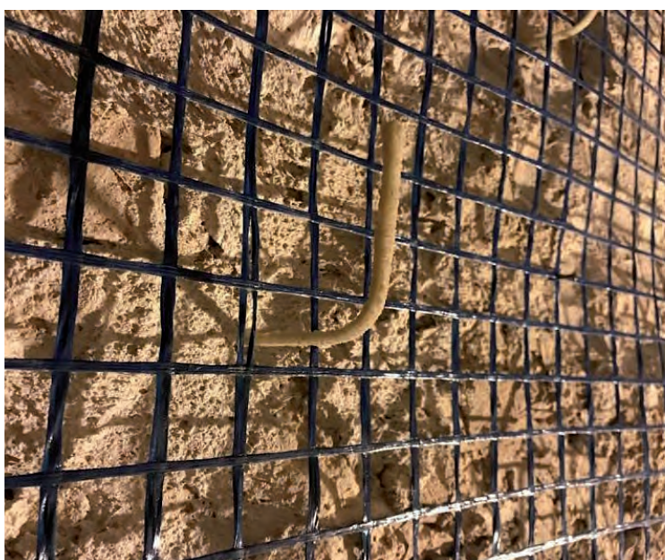
The masonry was strengthened with MAPE-ANTIQUÉ STRUTTURALE NHL and MAPENET EM40.
