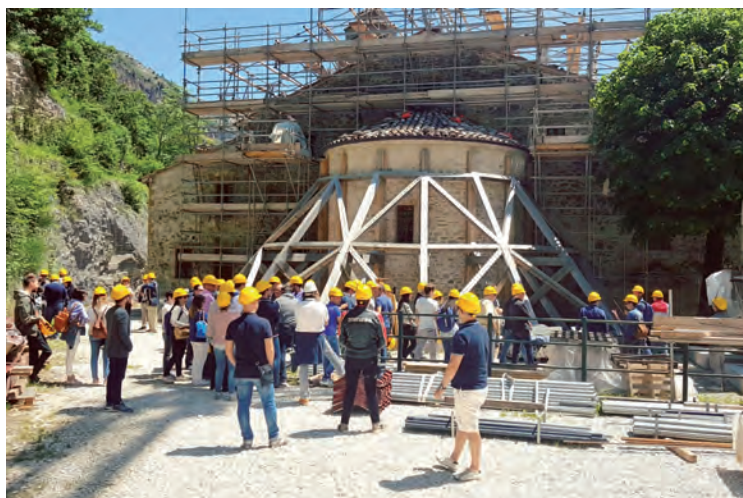
The FRP SYSTEM was used to strengthen the apse.
