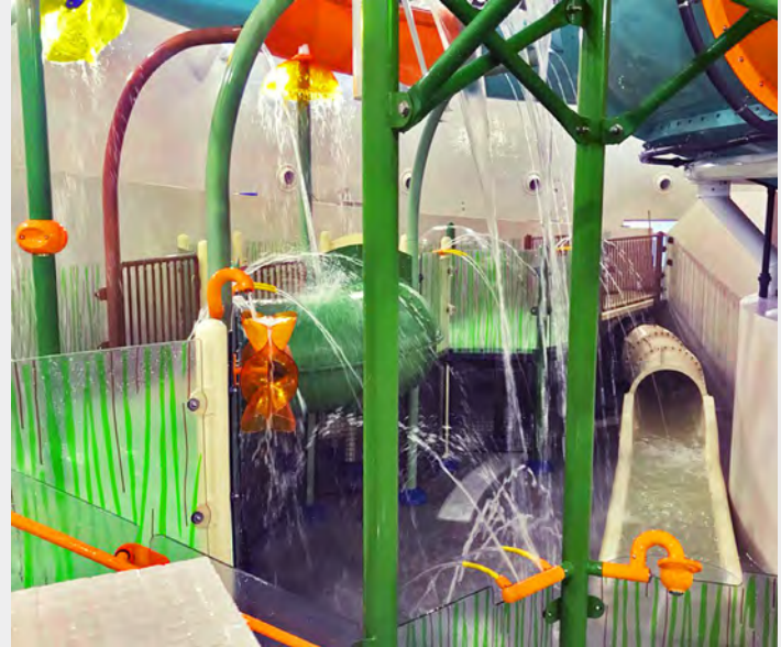
Preview of Vortex's family water attraction during final installation and testing at The Wave Coventry in the UK, winner of a World Waterpark Association Leading Edge Award.
